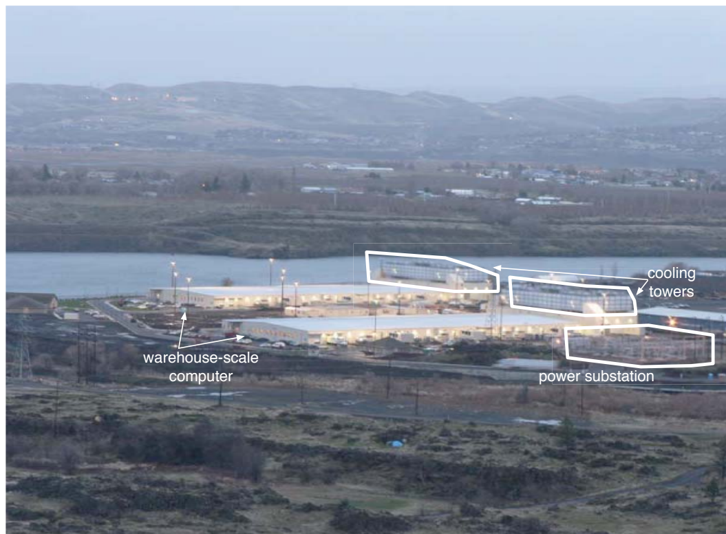
Figure 1.1: A datacenter with cooling infrastructure and power delivery highlighted.
