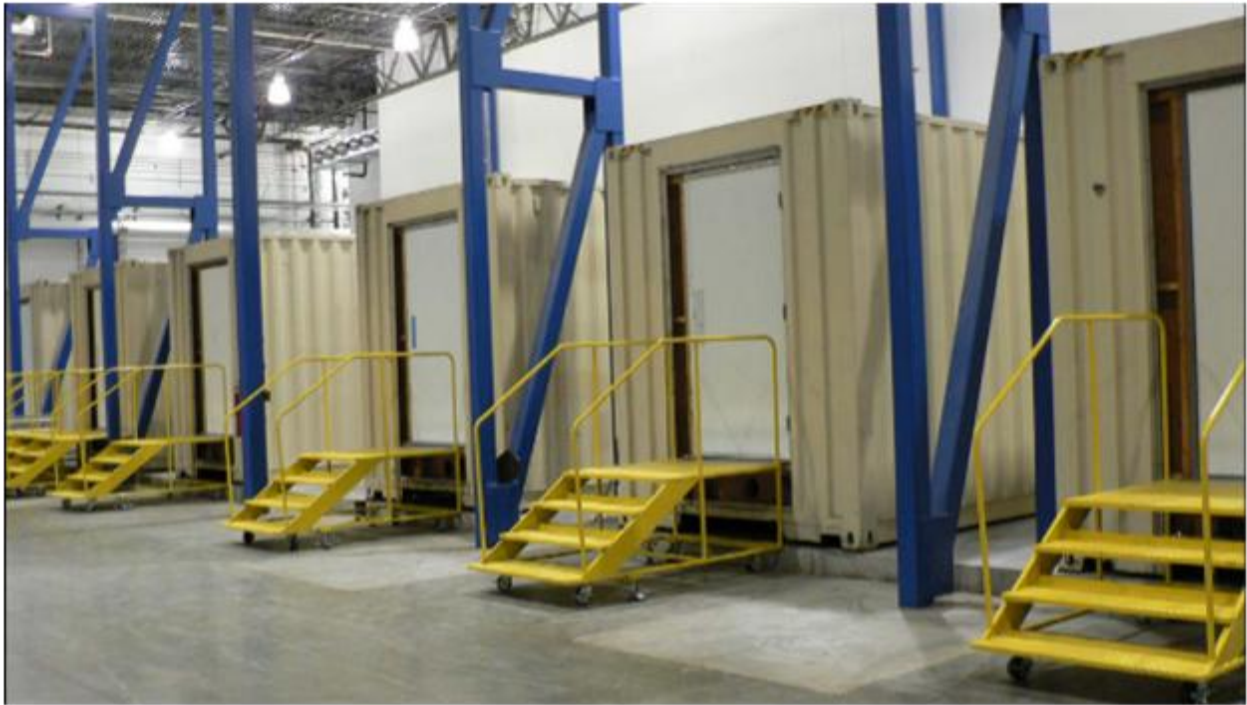
Figure 4-15: Google's container-based datacenter
